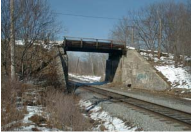
View south of Perkins Road Bridge over B&M Railroad
