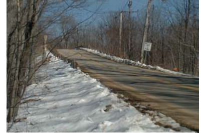
View east of limited site distance on Perkins Road Bridge
