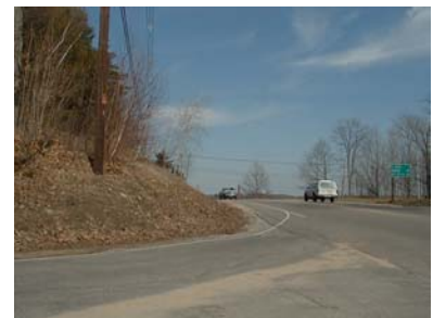
Limited visibility from Town Hall Road of oncoming Rte 155 traffic makes this an extremely dangerous intersection.
