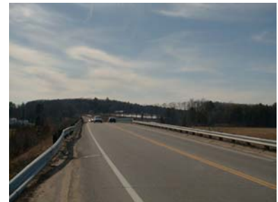
Picture 0 View of limited visibility from intersection of Pudding Hill Road looking west onto Route 155.
