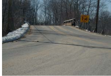
View west of limited sight distance and dangerous intersection at the Perkins Bridge/ Evans Road-Perkins Road split
