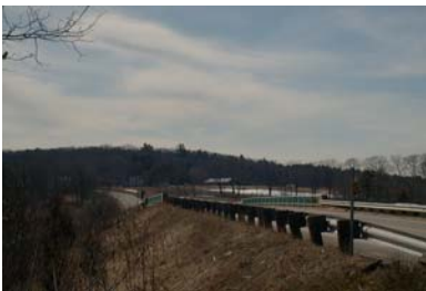
View west onto the Rte155/Knox Marsh Road Bridge of steep dip that makes for limited sight distance
