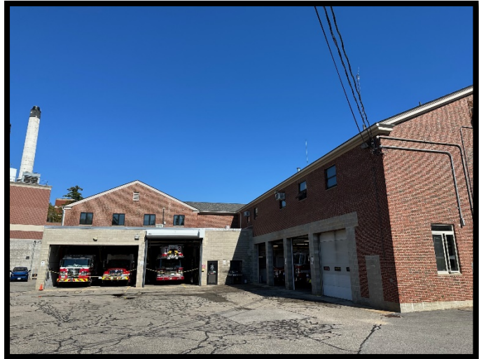
Figure 51 – Durham Fire Headquarters
