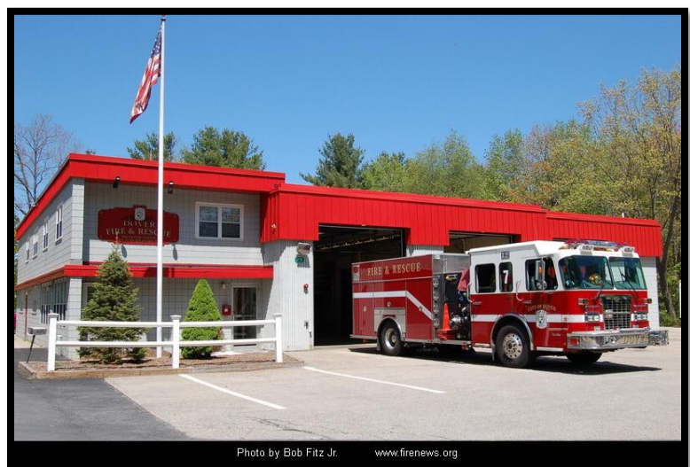
Figure 47 – Dover South End Fire Station
